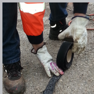
Roll BandFill onto the surface following the path of the crack
