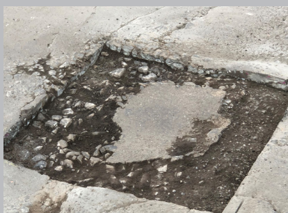
Easily repair damaged surfaces with a general depth of 25 – 60 mm.
