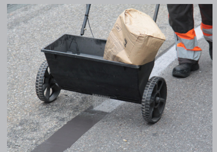
Add skid-resistance by applying glass grains over the still wet surface.
