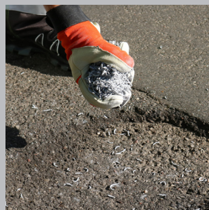
Apply an initial layer of maximum 15 mm.
