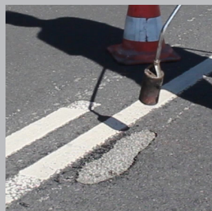
Remove moisture with a propane fueled heat torch.
