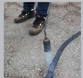
Sufficient heat has been applied when the material starts to bubble.
