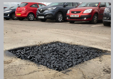
Rapid setting means that traffic can be re-opened within just 20 minutes.
