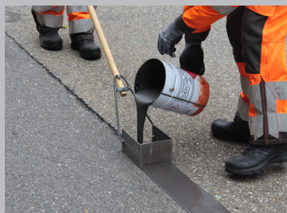
Use a screed box to apply the material across the repair area.
