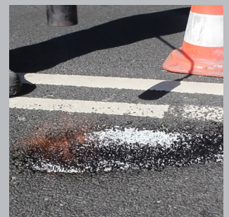
Heat material thoroughly and repeat process as necessary.
