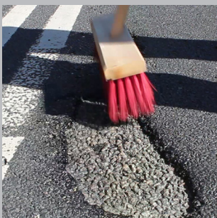
Remove debris and clean the repair area thoroughly.
