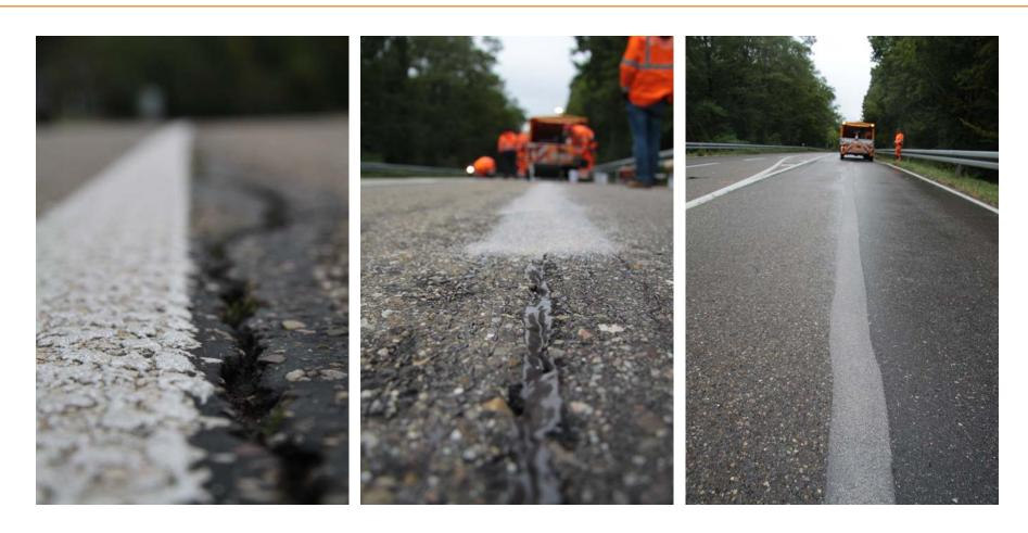
**ColdFill - mix, apply, dry.**Durable and quick repairs of long and irregular cracks!
