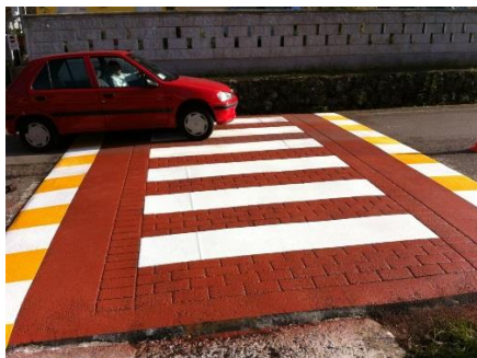
Highlighting a pedestrian crossing with red colored AquaRoute™ Deco Rough : application on stamped asphalt, combination with white and yellow PREMARK®
